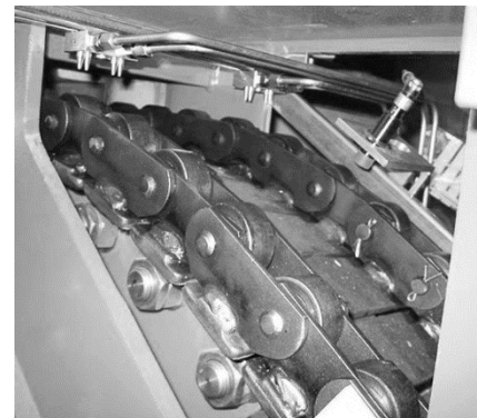
Escalator chain lubrication
